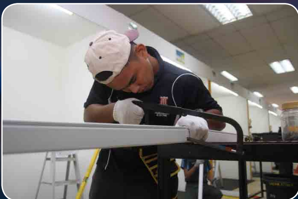
Junior Electrical Installation
