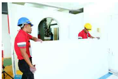
Drywall & Plastering Systems (Demo)
