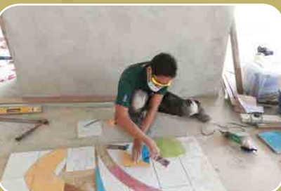
Wall & Floor Tiling
